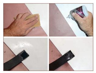
FIGURE 14-10: Gluing nylon straps to a styrene sheet with CA adhesive
