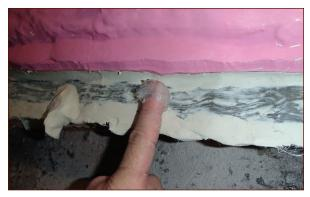
FIGURE 7-49: Applying petroleum jelly as a release agent. Icky.
